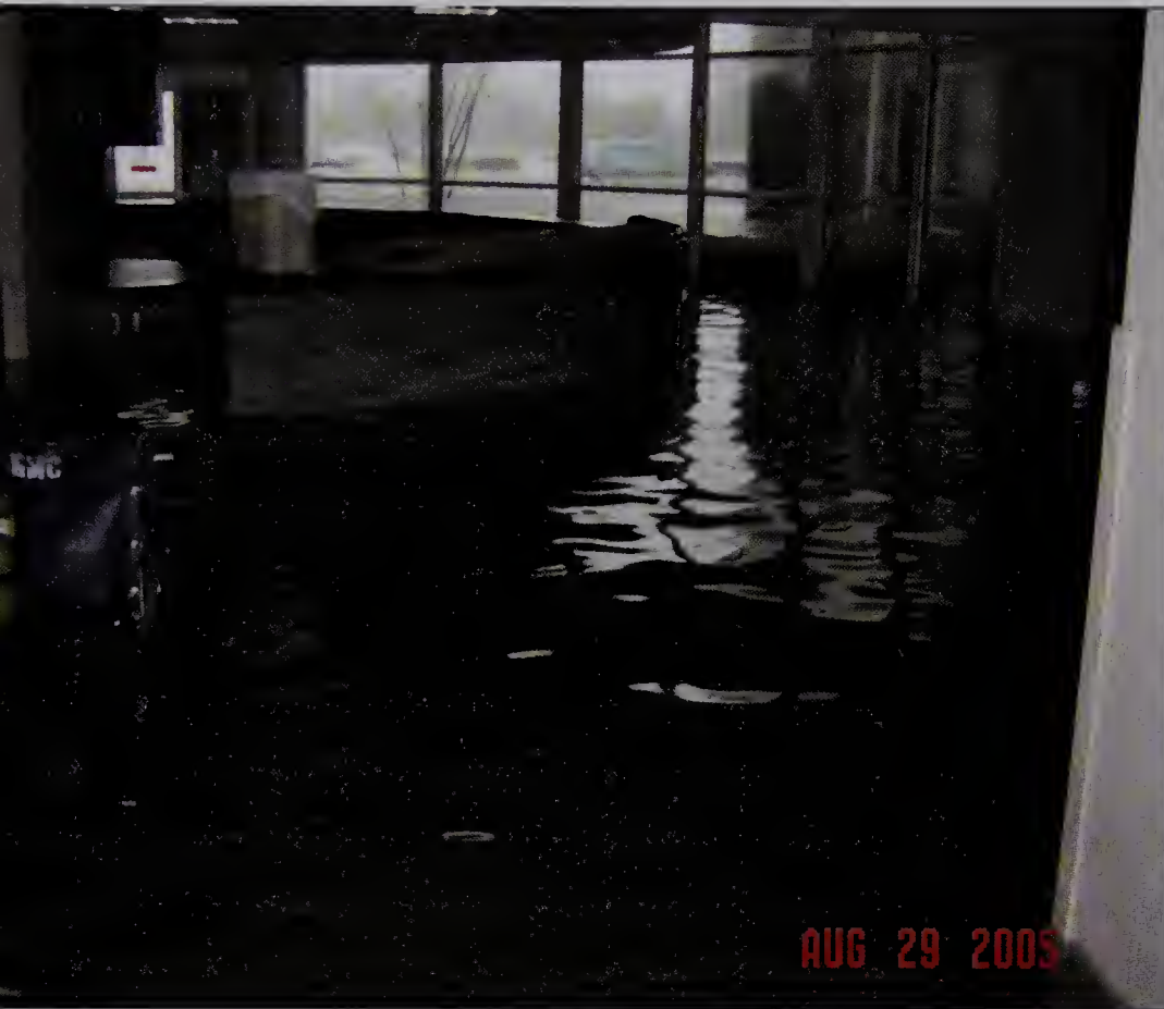
Flooded reception area, Hancock Medical Center, Mississippi Provided to Committee
